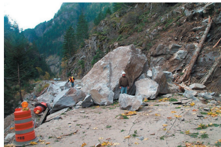
A rockslide on Highway 20 in Washington State cuts off access to Diablo, Wash., Sunday, November 9, 2003. The rockslide destroyed parts of the roadway and guardrail, and boulders and debris in excess of 100 tons, including a 50-ton boulder, blocked both highway lanes. (Washington State Department of Transportation photo)
