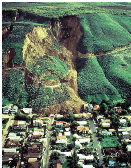
Homes lie damaged under this large earth flow in LaConchita, Calif., Saturday, March 4, 1995. On January 10, 2005, a portion of this area became a debris flow during heavy rain, destroying several homes and killing 10 people. (USGS photo/Robert L. Schuster)
