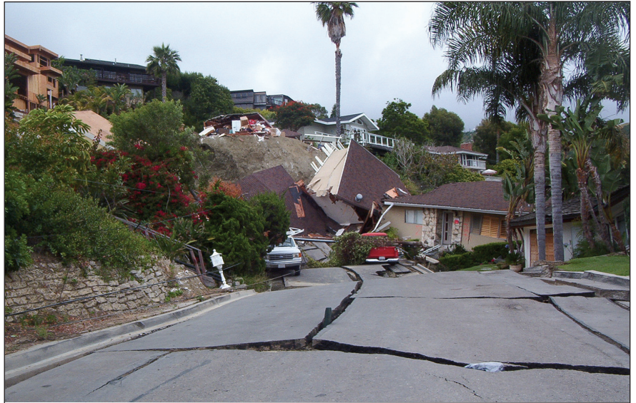
Bluebird Canyon landslide, June 1, 2005, near Laguna Beach, California. This area experienced a landslide in 1978, about 50–100 meters (150–300 feet) to the west of the 2005 event. The 2005 landslide caused 350 homes to be evacuated, of which 15 were damaged or destroyed. The movement was most likely caused by heavy rains in January and February 2005. This type of deep-seated landslide movement is common in southern California in the months following a season of heavy rainfall. Photograph by Jim Bowers, USGS.
