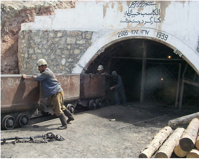
Figure 2. Karkar Mine, Baghlan Province. This North Coal Department mine, owned and operated by the Afghan government, is currently operating far below prewar (1978) capacity. The mine ventilation system is no longer fully functional, electric railcars have been replaced by winches, and expensive imported timbers are being used for roof support in place of local materials, which are no longer available.
