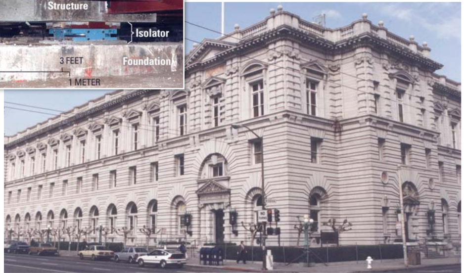
The 100-year-old Court of Appeals Building in San Francisco, California was retrofitted after the 1989 Loma Prieta earthquake using base-isolation technology (inset) and was fully reoccupied in 1996. Base-isolation systems dampen the shaking energy fed into the structure through its foundation, thus reducing the likelihood of damage. Sensors placed below and above the isolators allow measurement of the effectiveness of the system.
