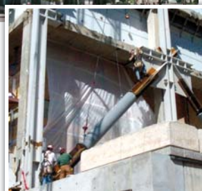
The Bennett Federal Office Building in Salt Lake City, Utah, built in 1965, underwent a major seismic retrofit completed in 2003. To reduce the shaking in the structure during strong earthquakes, the building was fitted with novel, unbonded diagonal braces and dampers (inset). Sensors have been deployed throughout the building to validate the expected improvement in seismic performance of the building during strong tremors. Red arrows indicate the locations of the sensors and show the 26 components, or directions, of motion that the sensors record.
