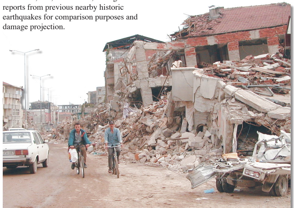
Photograph showing destruction caused by the 1999 Izmit, Turkey, earthquake. For events such as this, PAGER will provide emergency relief organizations with a rapid assessment of an earthquake's impact that will allow them to determine which areas require the most attention.
