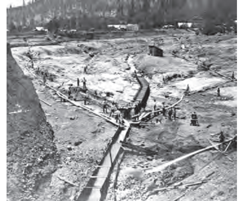
Figure 2. Gravel deposits were washed into sluices (from center to lower part of figure) where gold was recovered.
