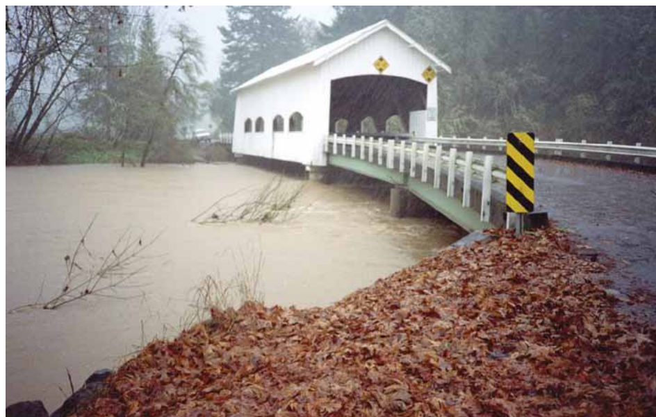
Flooding on November 19, 1996 on the Calapooya River at the Rochester Bridge located on County Road 10-A near Sutherlin. (Photograph courtesy of Douglas County Department of Public Works, Roseburg, Oregon.)
