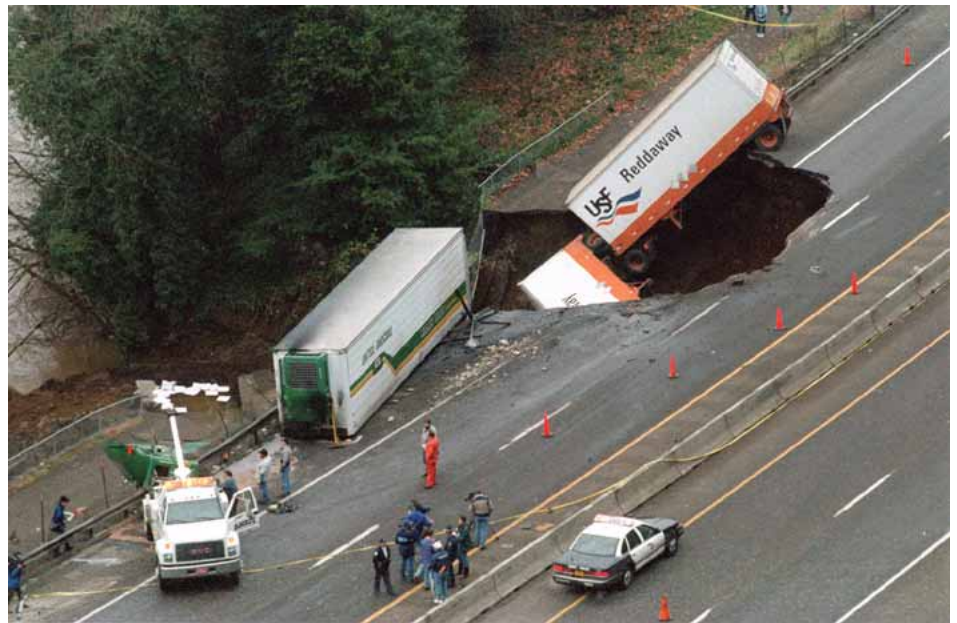
A mudslide on November 21, 1996, resulted in the collapse of a section of Interstate 5 along the South Umpqua River near Roseburg, Oregon. Damage to roads and bridges was widespread during the storms of November–January 1996–97. (Photograph by Christian Murdock, Roseburg, Oregon, News Review; used by permission.)
