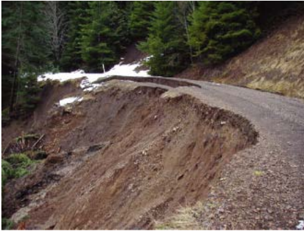
Heavy rain in December 2001 triggered a road failure on a tributary of Blowout Creek. The resulting debris flow caused increased turbidity at the monitoring station for several days.
