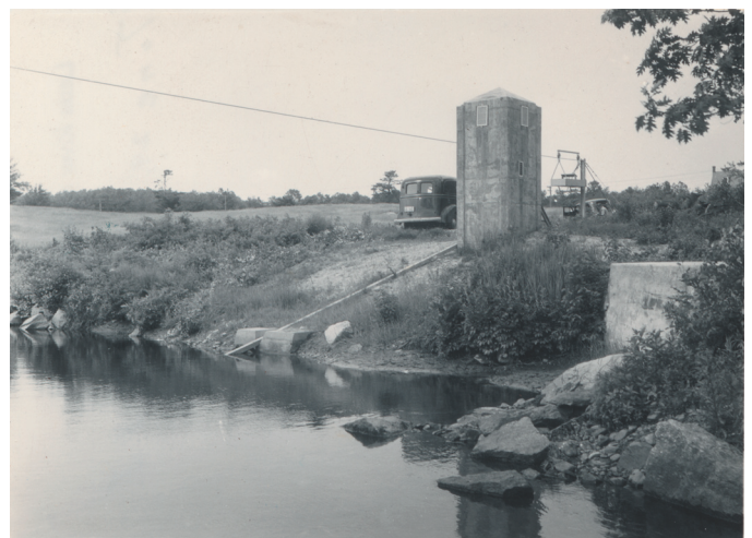
Streamflow-gaging station Little River at Oxford, Massachusetts. This 1940 photo shows the gage house, cable car, and cableway.
