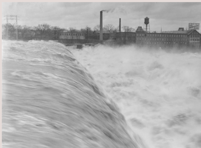
The Connecticut River at the Holyoke Dam, Holyoke, Massachusetts, March 1936. The highest discharge ever recorded at the Montague City station, 236,000 cubic feet per second, and the highest stage, 49.2 feet, were recorded during the flood on March 19.
