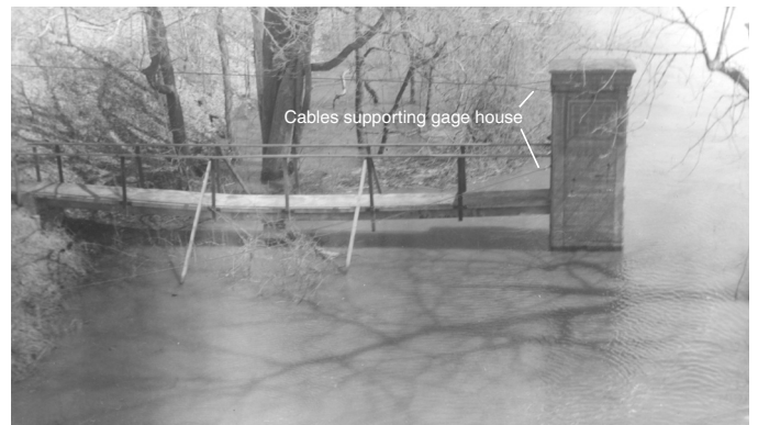
Figure 4. The Montague City station under high water, April 6, 1960. Recorded stage was 37.50 feet.
