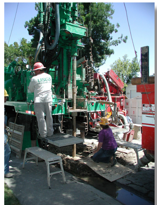
Figure 3. Drilling a monitoring well in Modesto, California.
