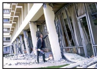
The 1971 San Fernando, California, earthquake (magnitude 6.7) severely damaged the recently built Olive View Hospital. This building was not instrumented with seismic sensors. Accordingly, no data were obtained to understand how the damage initiated and progressed during the intense shaking. The building was razed and replaced with a stronger structure that survived the 1994 Northridge earthquake (see back page).
