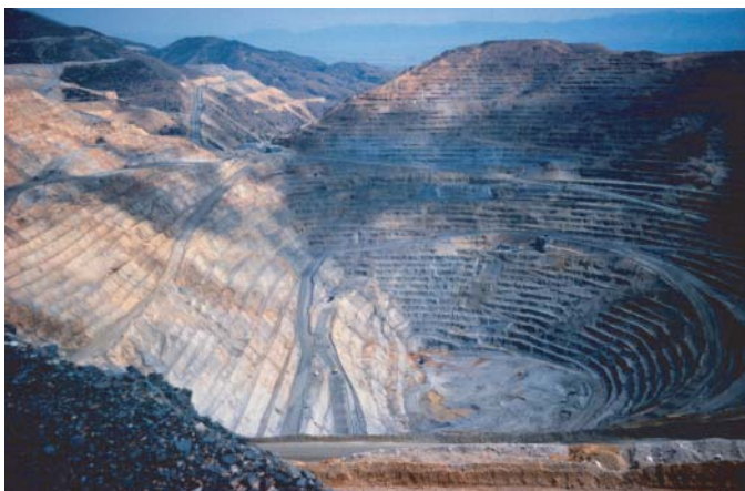
Figure 1. Bingham Canyon porphyry copper deposit, Utah. The pit is about 3 kilometers across and has produced nearly 12 million tons of copper since it opened in 1904. Photograph by Charles Cunningham, U.S. Geological Survey.
