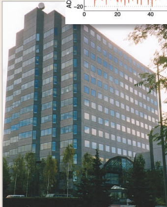
During the fall 2002 magnitude 7.9 Alaska earthquake, shaking monitors in this 14-story building in Anchorage recorded complex twisting and swaying motions. When analyzed, these records (including that shown above taken on the building's roof) will help engineers improve building designs.
