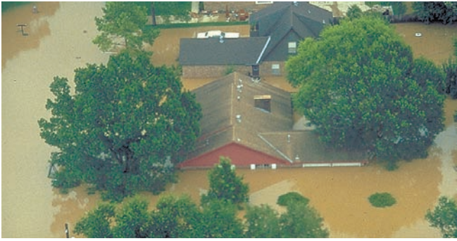
Figure 4. Land subsidence of 5 to 7 feet in a residential area in northern Houston exacerbated flooding in June 1989.
