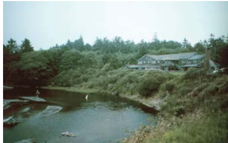
Figure 4. Kalaloch Lodge in Olympic National Park, Wash., is threatened by erosion. Long-term plans call for moving the lodge back from the cliff edge. Photograph by Erika Hammar-Klose, USGS.
