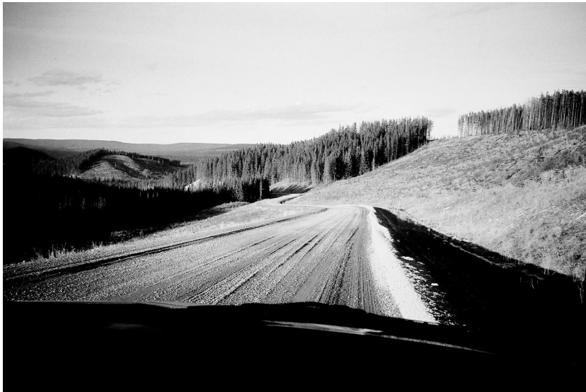
Photo No. 2: Mainline Road (5 November 2002)
