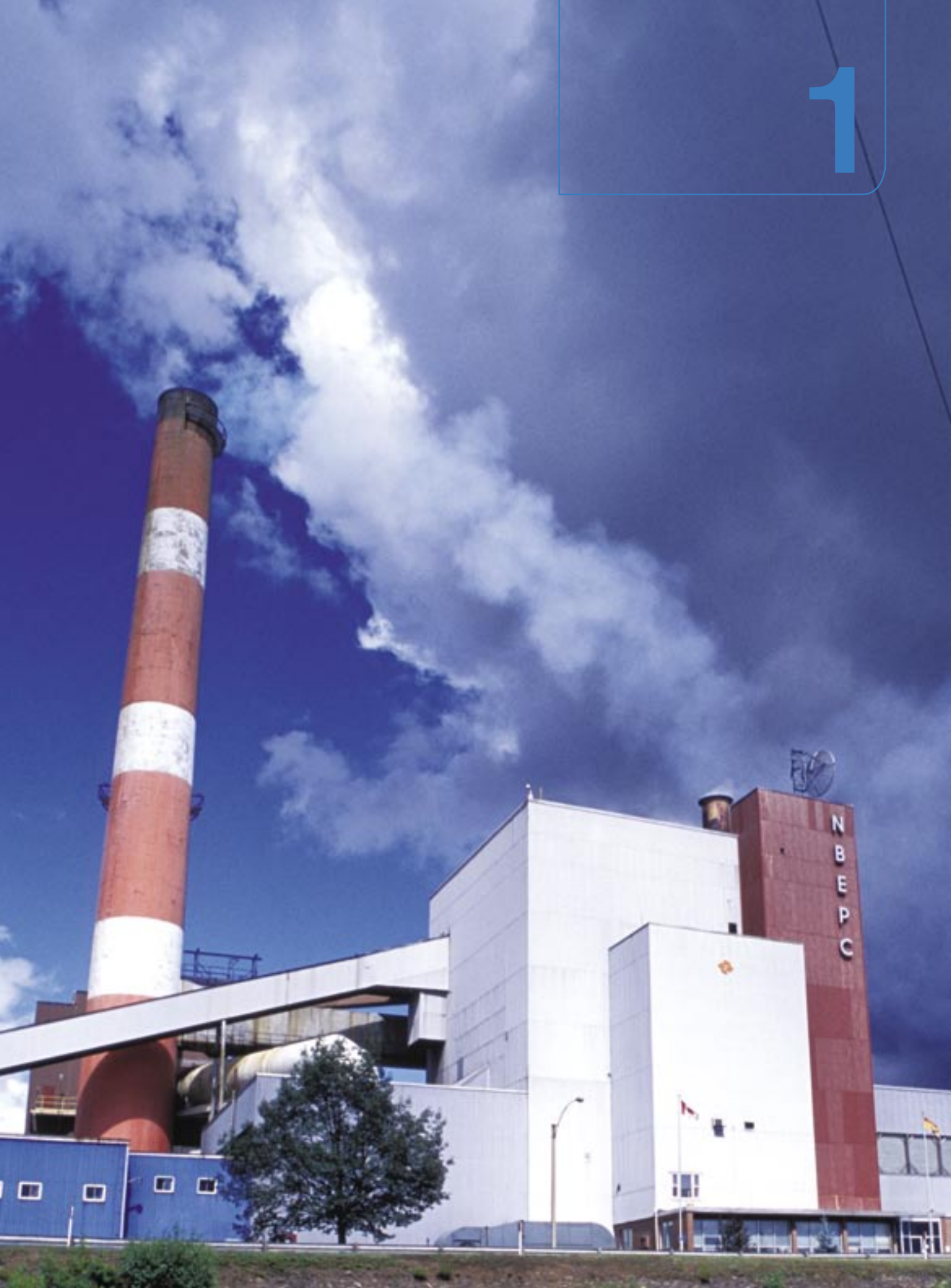
GRAND LAKE fuel used coal, capacity 57 MW, location New Castle Creek, New Brunswick
