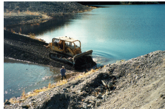
Cover soil is replaced from a stockpile or a new location about to be mined
