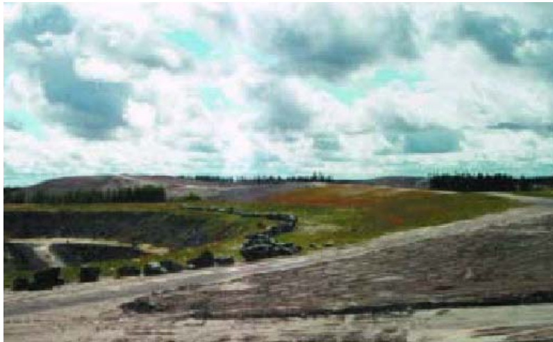
Detour Mine - Foreground – open pit safety berm; Background – resloped and revegetated waste rock piles
