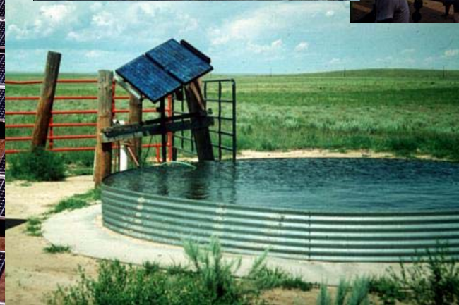
PV-powered water pumping
