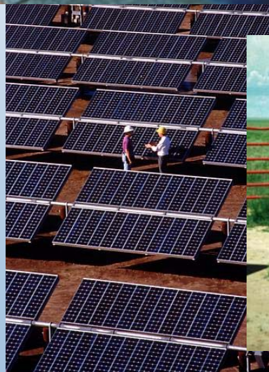
210 kW PV system at SMUD's Hedge substation
