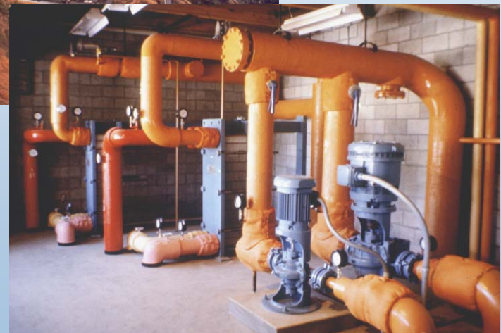
Heat exchangers and circulation pumps
