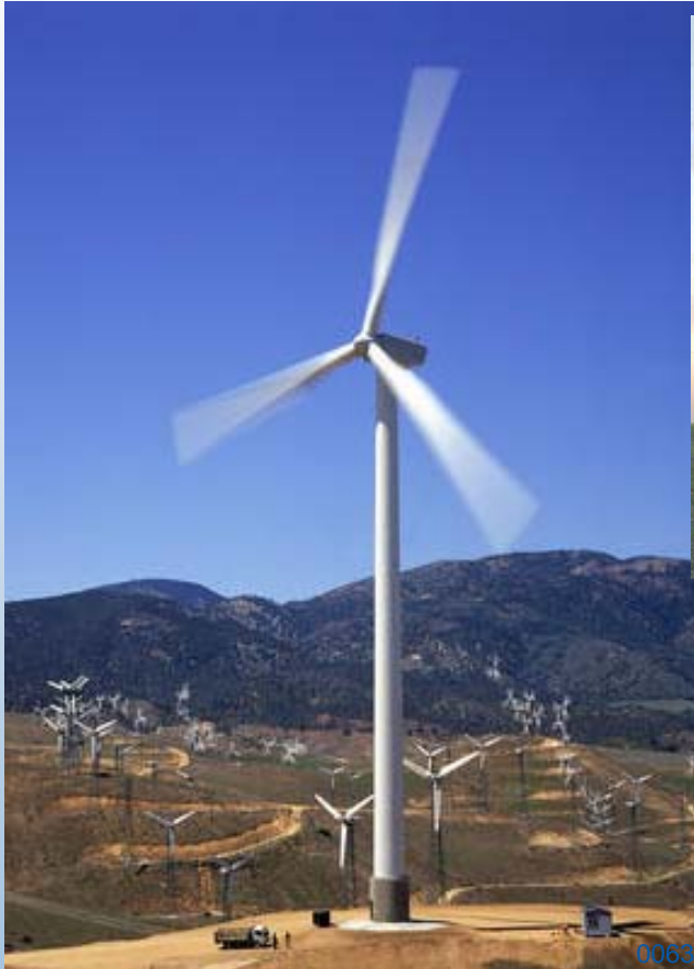
GE Wind's 1.5 megawatt wind turbine installed in Tehachapi, California
