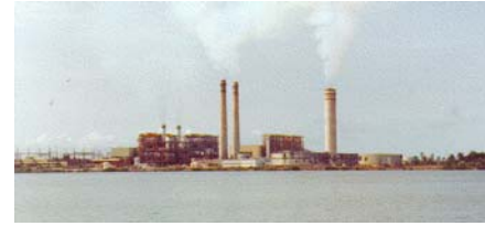
Central generating station
