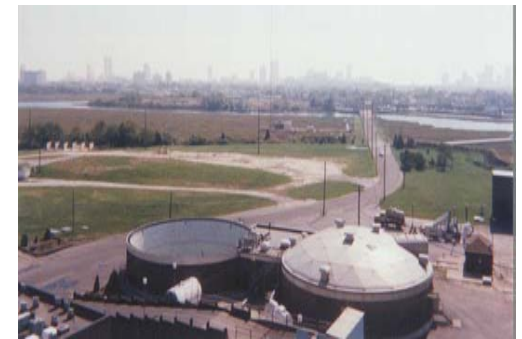
The 7.5-MW Jersey Atlantic Project Atlantic City, NJ Expected On-Line Spring 2004
