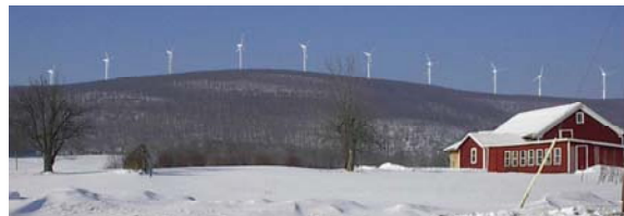
The 61-MW Pocono Wind Farm Northeast of Scranton, PA Expected On-Line Fall 2003
