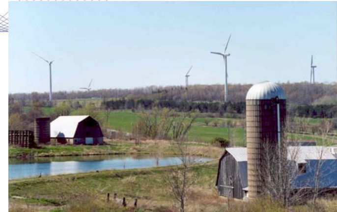
The 31-MW Fenner Wind Farm Madison County, NY On-Line June 2002
