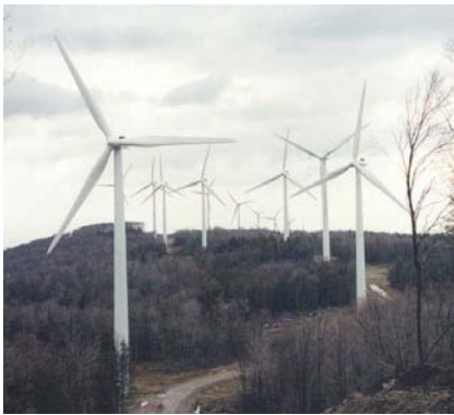
The 66-MW Mountaineer Project Allegheny Plateau, WV On-Line December 2002
