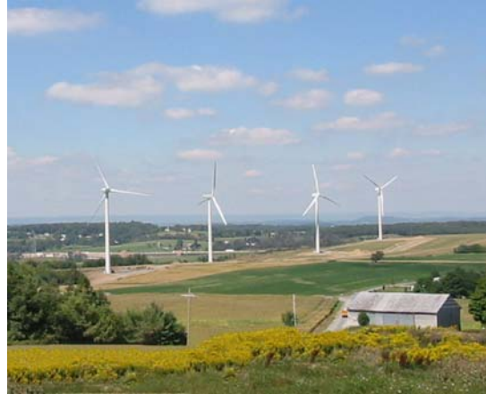
The 9-MW Somerset Wind Farm Visible From the PA Turnpike On-Line October 2001
