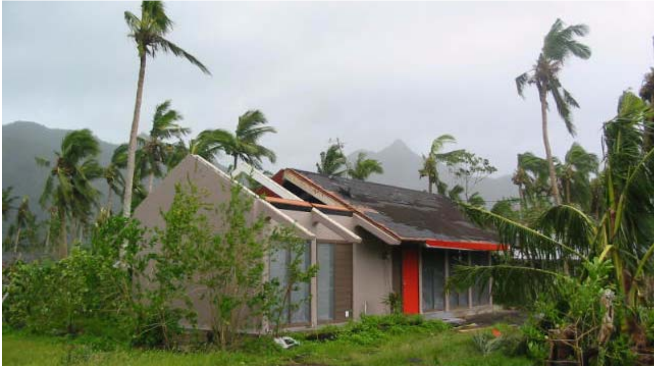
Figure 1.4. The next house down from the two CMDL staff houses in Tafuna. The occupants were sheltering in the bedroom when the roof was blown off above them. The CMDL houses fared better.
