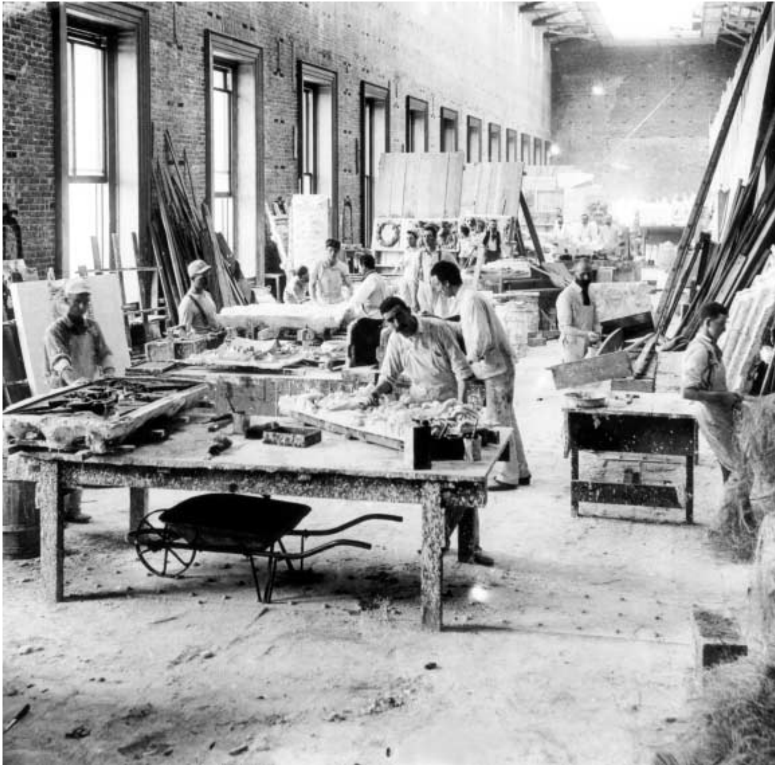
The construction staff established a large modeling shop on the building's second floor so workers could carry out artists' designs in plaster, July 19, 1894.
