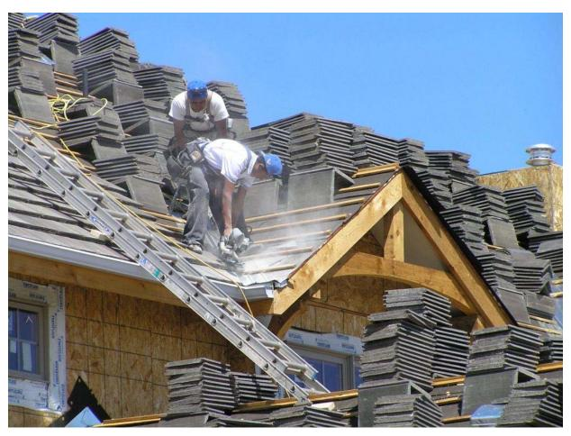
Figure 3. Roof arrangement while installing tiles.
