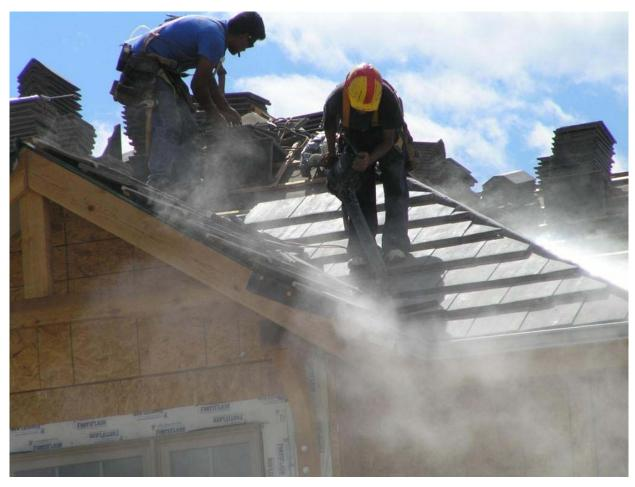
Figure 4. Workers using leaf blower to clean dust from tiles.
