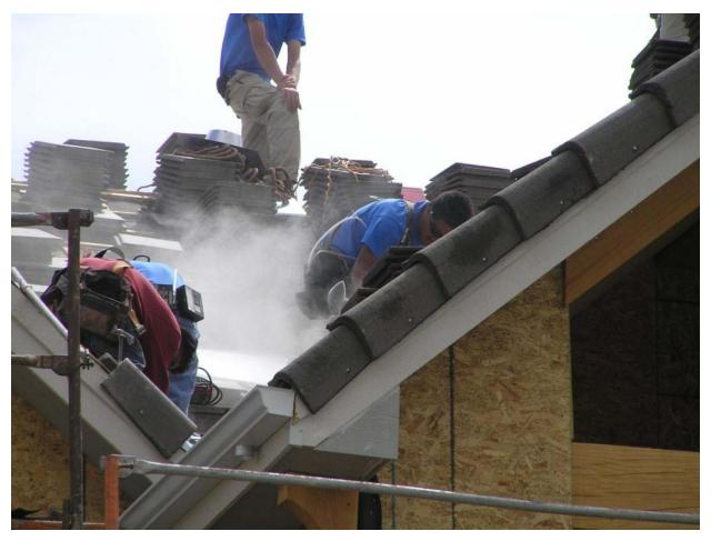
Figure 5. Workers cutting concrete roofing tiles.
