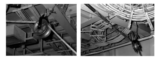
Figures 14a and 14b. Sheaves for Cable Pulling
