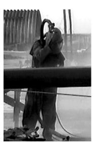
Figure 1. Abrasive Blaster Blasting Material Above Waist Height
