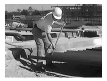
Figure 2. Gator Bar Worker Positioning Angle Iron
