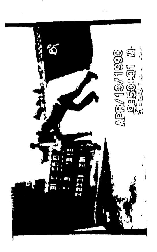
Figure A14 Deliveryman pushing loaded 4-wheel hand truck (approximately 680 lbs - includes weight of band significant stress to the back, and increase chances for slip and fall injuries if the foot and ground truck) up 6 degrue rank to store service entrance (Gomment Pushing or pulling loads up ramps cause contact is not good Longer, lower grades are recommended over short, steep grades ]
