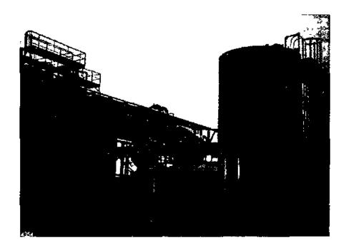
Figure 14. MO-2 methanol storage tanks. Note dike around both tanks.
