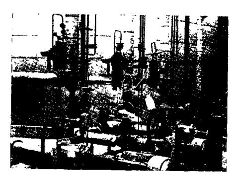
Figure 24. Storage tank recirculation pumps with double mechanical seals.
