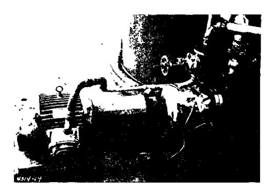
Figure 33. Second spray tower pump; wrapped; tubes in place.
