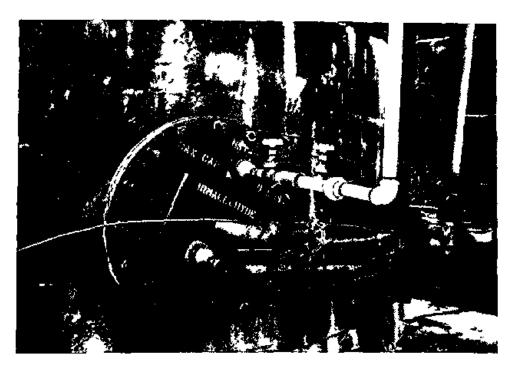
Figure 23. Formaldehyde storage tank manhole with steam lines attached.
