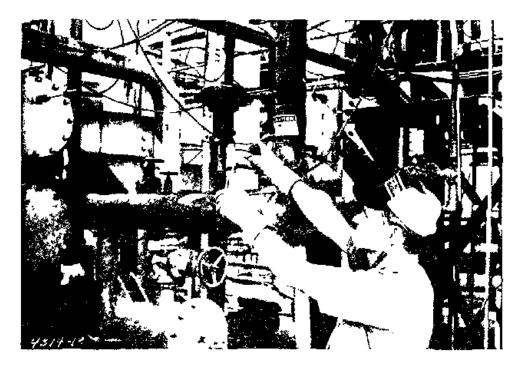
Figure 5 Process sampling at absorber/heat exchanger by operator.
