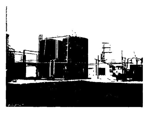
Figure 22. Formaldehyde storage and loading area. Can see scrubber on left of formaldehyde storage (bottom).
