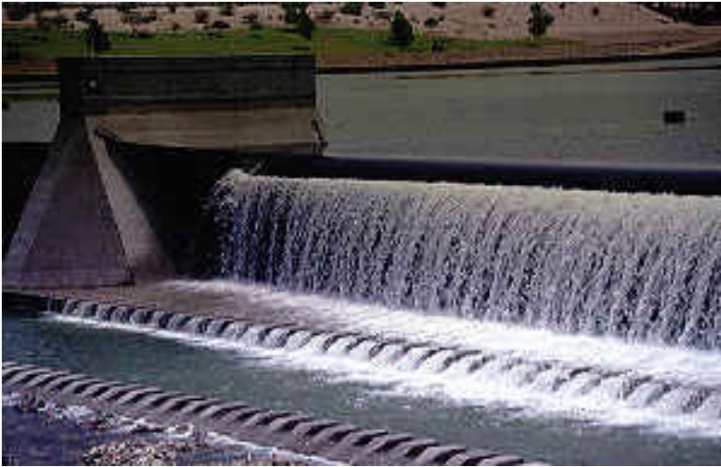
Water spilling over one of the rubber dams.
