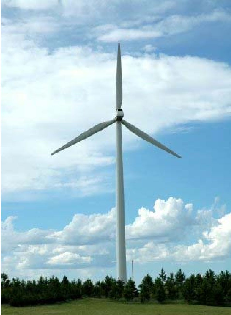
Rosebud's 750 kW Turbine produces 2.4 Mil kWh/yr.
