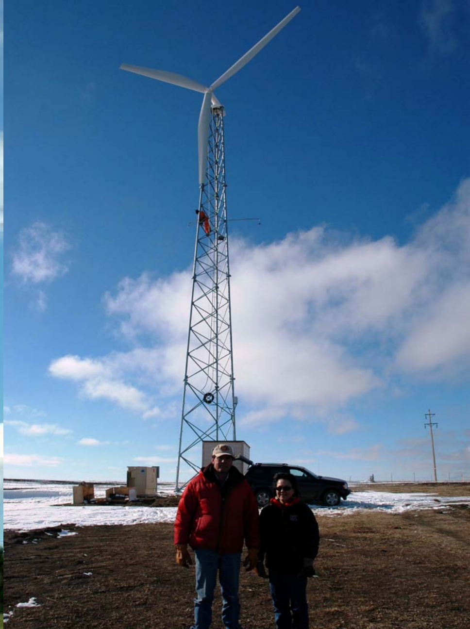
Ft. Berthold's 65 kW Turbine installed Sept 30, 2005
