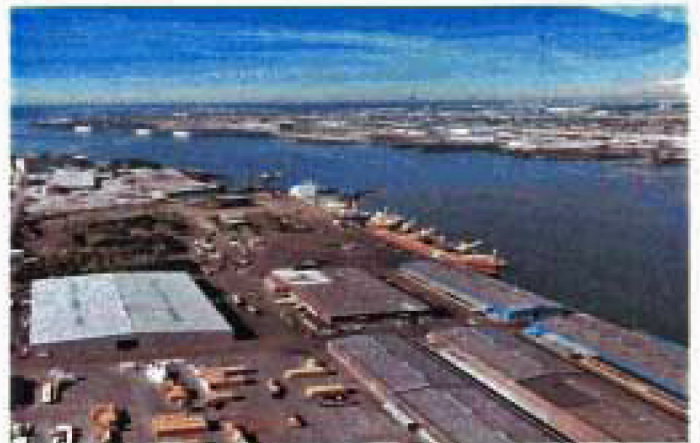
Beckett Street Terminal (NJ)
