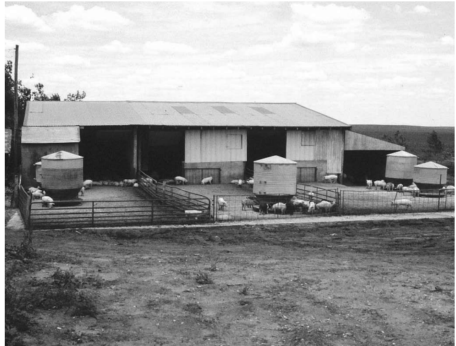
Figure 1.1. Muddy lots were being replaced with concrete. (APHIS photo by Lowell Anderson)
