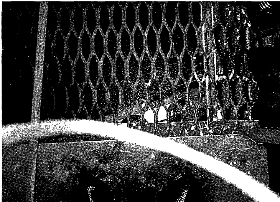
A walkway directly above the bean-canning line at the same firm. Although it is partially covered with sheet metal, most of the walkway is open allowing foreign matter to drop into the cans as people walk on it.
