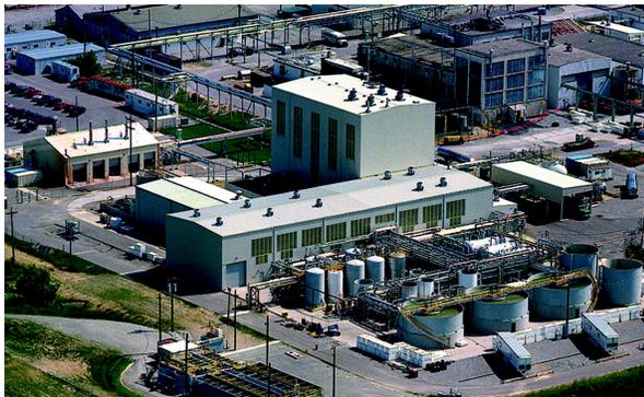
sites that made nuclear weapons. The site was designed as a large-scale, integrated facility capable of converting uranium ore and recycled material into uranium metal through a series of chemical and metallurgical conversions.
