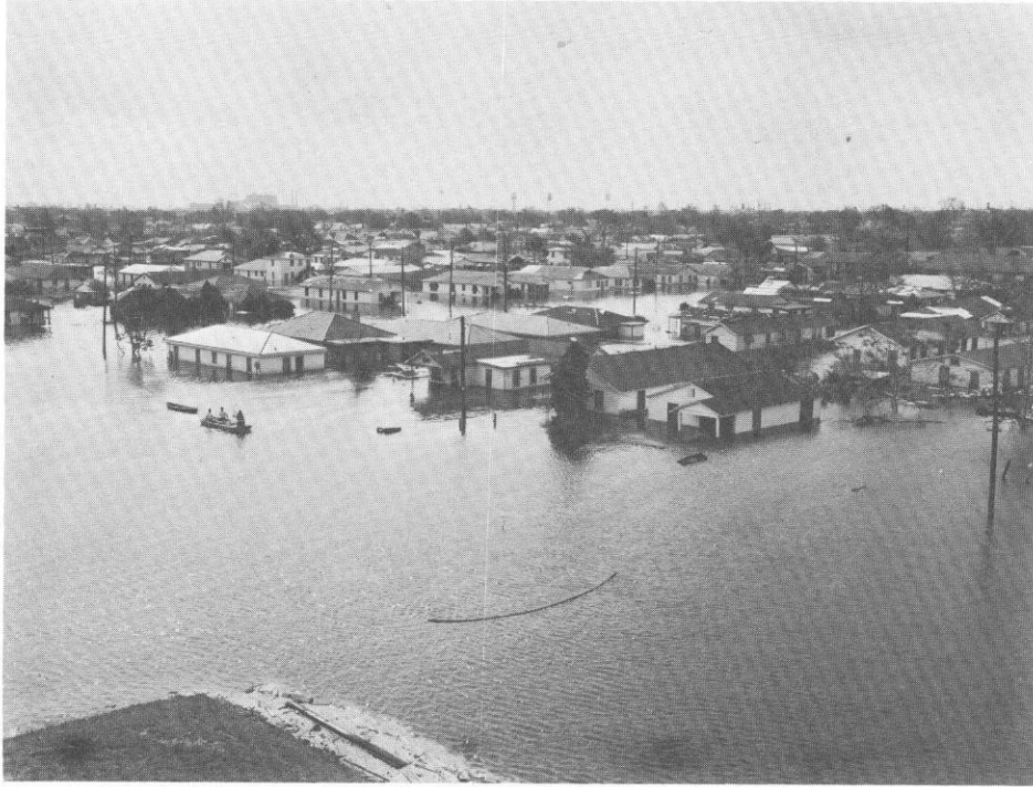
HIGH TIDE FLOODING EAST OF INNER HARBOR NAVIGATION CANAL NEW ORLEANS, LA., 11 SEPTEMBER 1965
