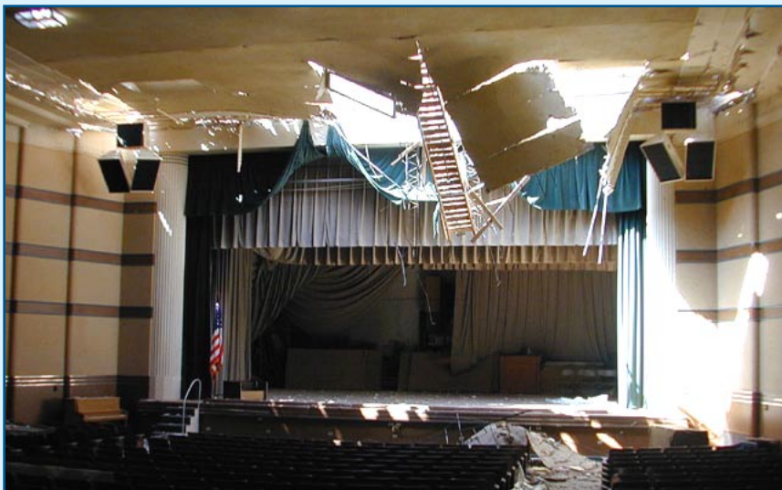
The tornado caused serious damage to Hoisington High School. Part of the roof structure was removed by the high winds.
