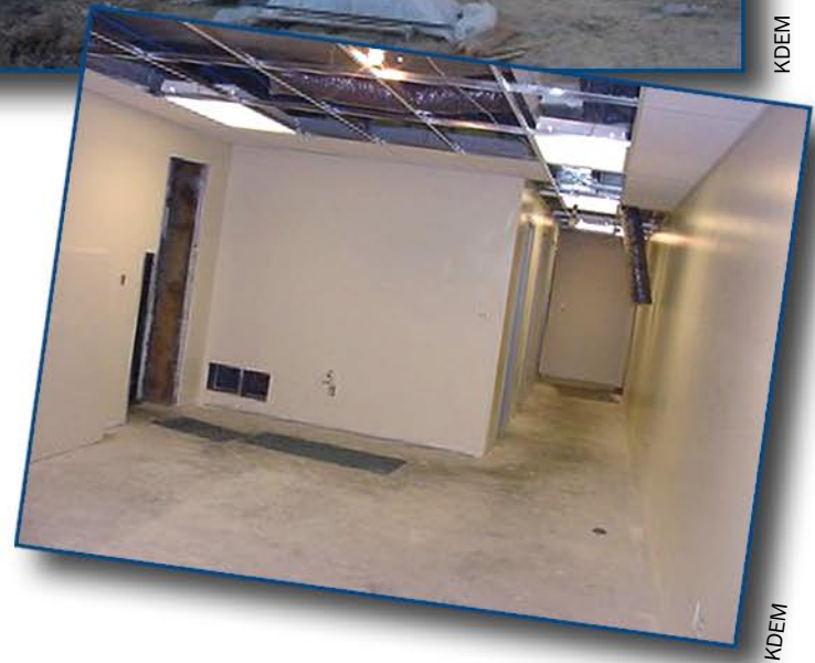
Construction of the reinforced ICF exterior wall at the rear of the shelter (top). Interior walls of shelter with gypsum board finish (bottom).
