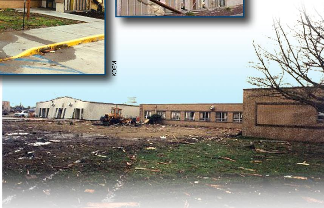
Rear view of damaged clinic building (left) and main hospital building (right).
