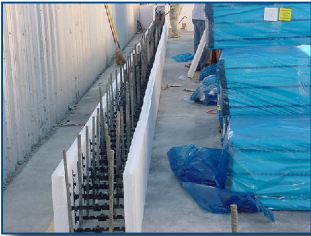
All perimeter walls were constructed with insulating concrete forms and reinforced with #5 bars spaced 8 inches on center to resist 250 mph wind speeds.
