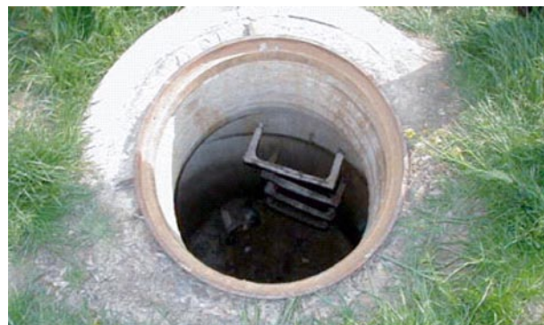
Figure 4-1. Landfill manhole where fatality occurred
