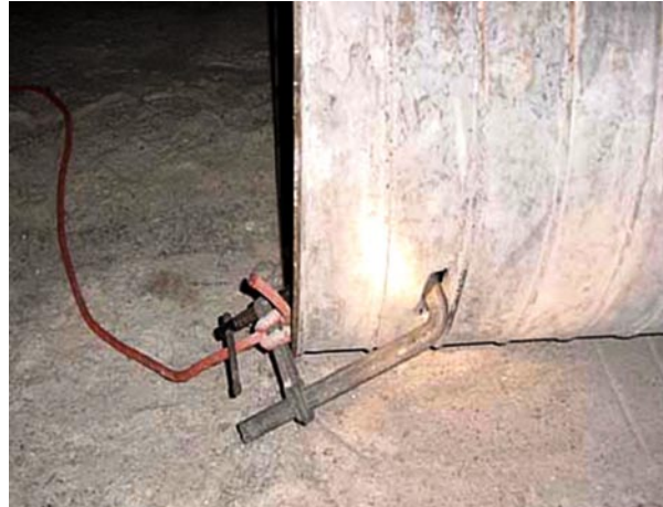
Figure 2-2. C-clamp attached to vent line
