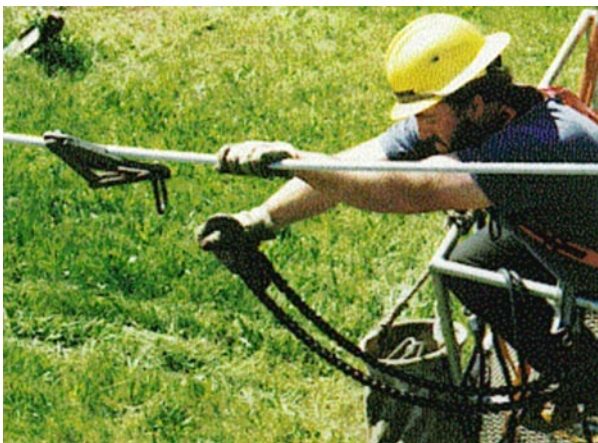
Figure 3-4. Reenactment of lineman removing gripper from conductor
