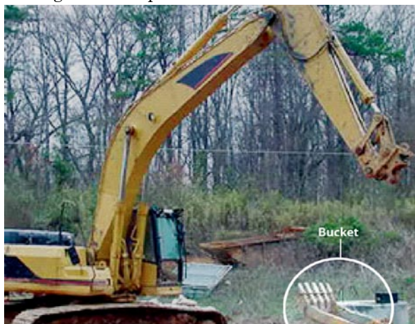
Figure 3-3. Excavator and dropped bucket
