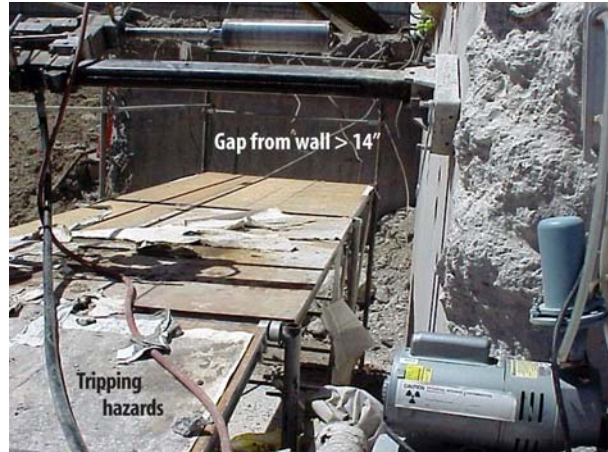
Figure 1-2. Scaffold deficiencies
