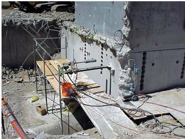
Figure 1-1. Scaffolding used during core drilling
