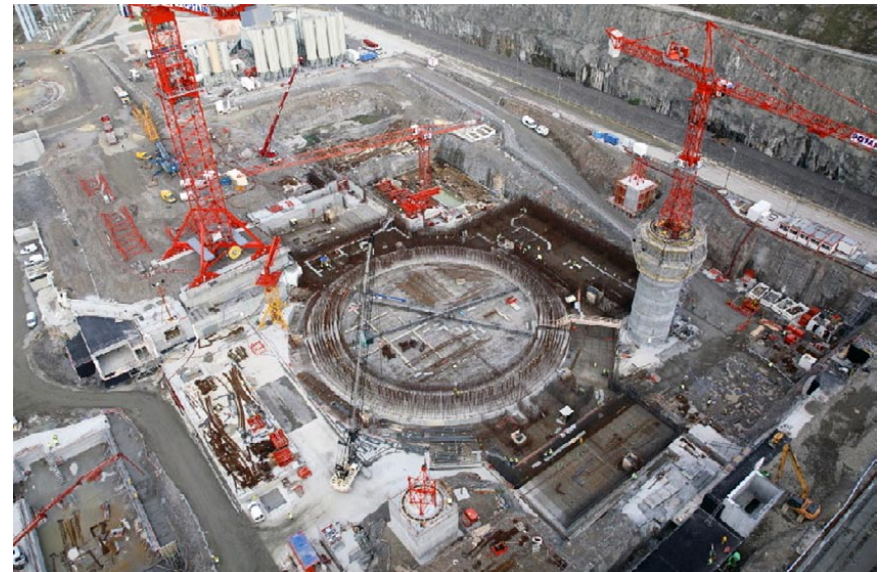
Figure 1-3. Flamanville 3 construction site and circular basemat for reactor containment
