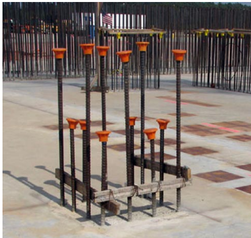
Figure 1-2. Concrete mat and rebar installation during construction of MFFF
