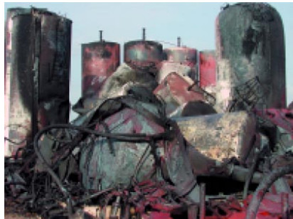
Figure 2-2. Melted storage tanks post-fire
