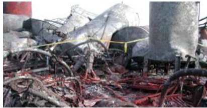
Figure 2-1. Collapsed blending tanks
