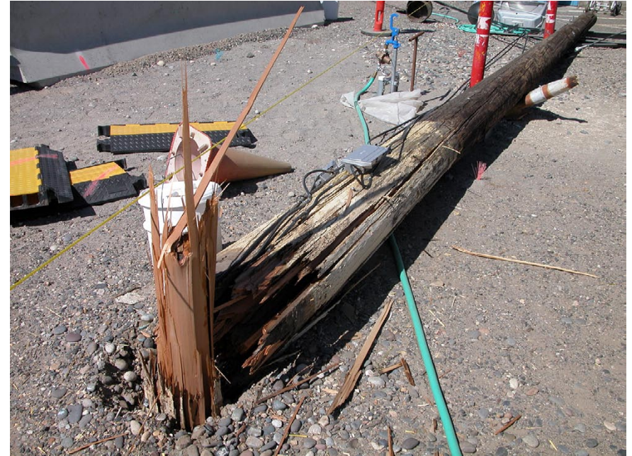
Figure 1-2. Snapped off utility pole
