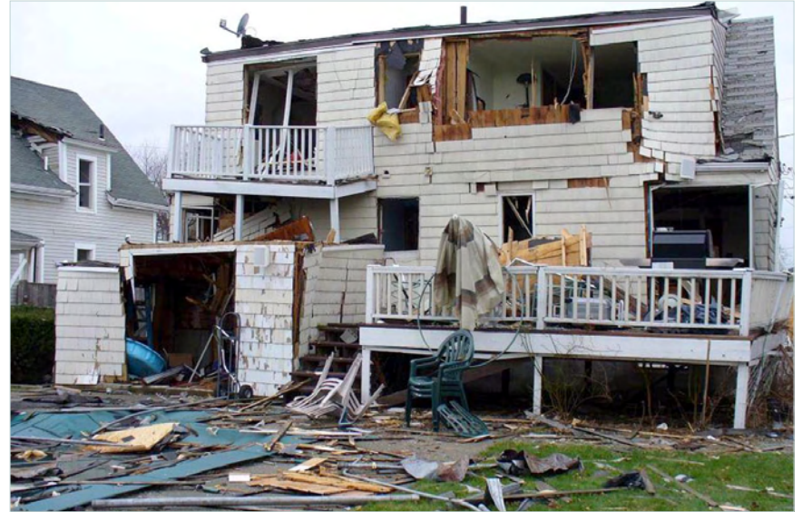
Figure 1-1. Nearby home destroyed in CAI explosion
