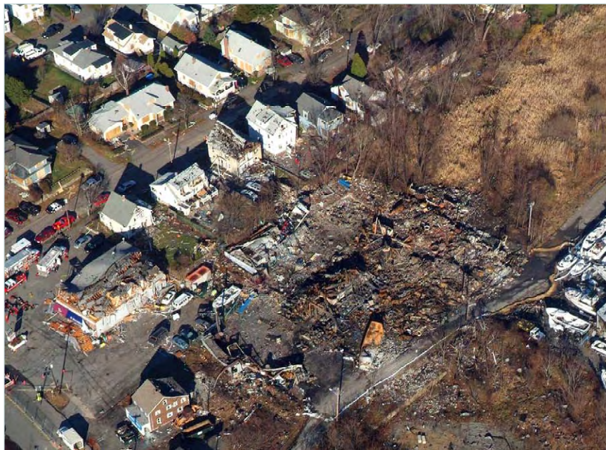
Figure 1-2. Aftermath of explosion
