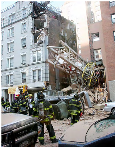
Figure 1-5. Collapsed crane protruding from building after March 15, 2008, accident
