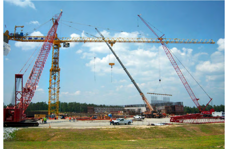
Figure 1-1. SRS cranes at MOX Project (yellow tower crane was shut down)
