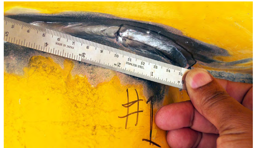
Figure 1-2. Cracks on turntable of SRS tower crane
