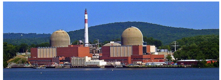
Figure 2-1. Indian Point Power Plant
