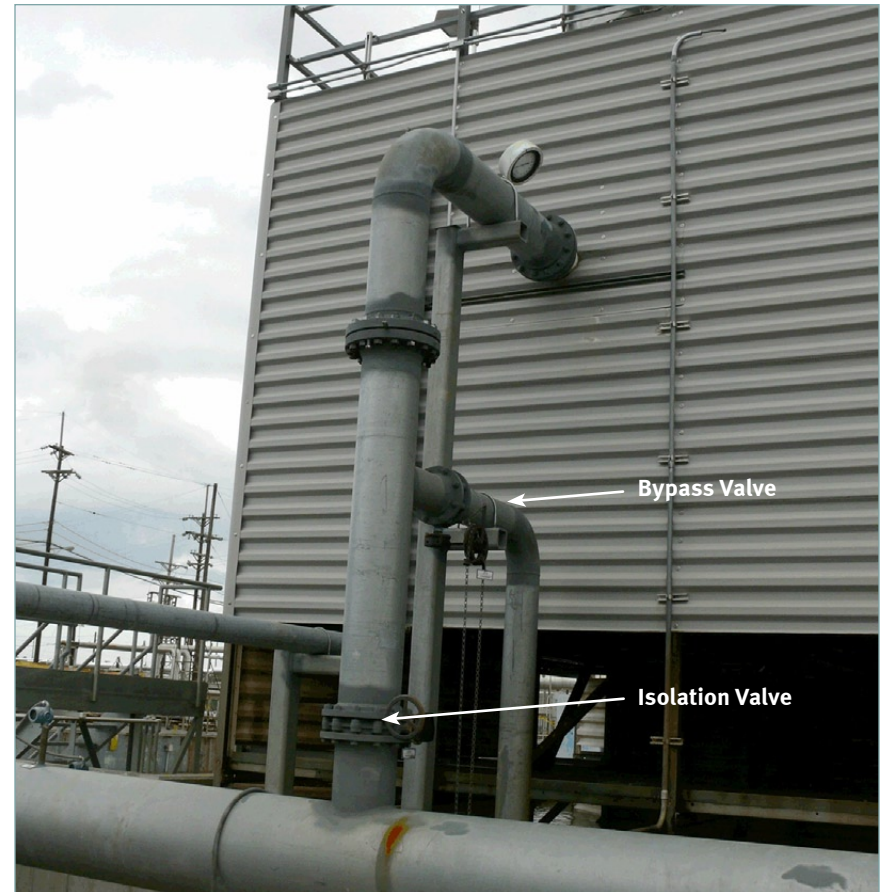
Figure 2-1. Cooling tower and piping arrangement
