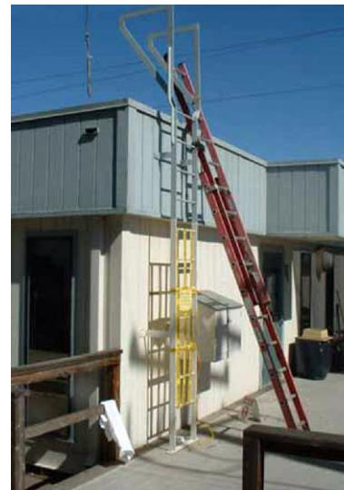
Figure 1-2. Accident scene showing the fixed ladder and an extension ladder added post-accident for temporary roof access
