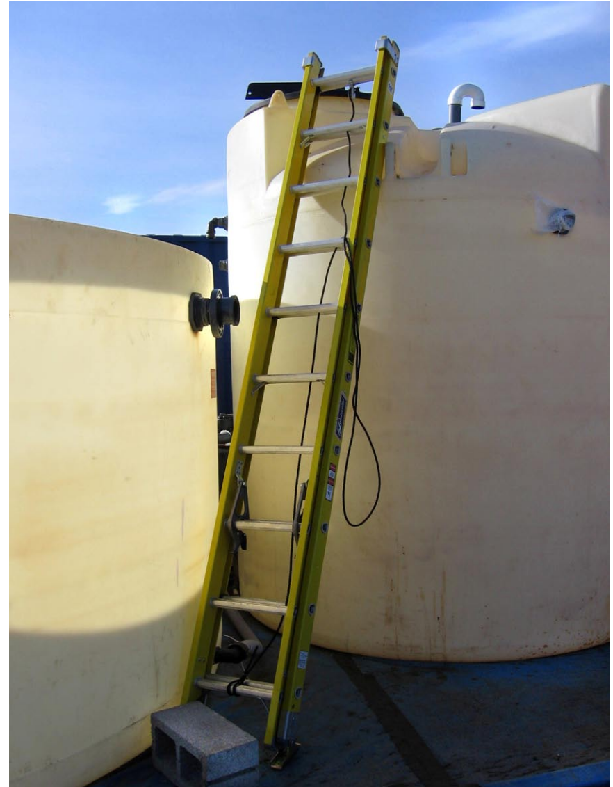
Figure 1-1. Tank and extension ladder (the worker fell into the tank on the left)
