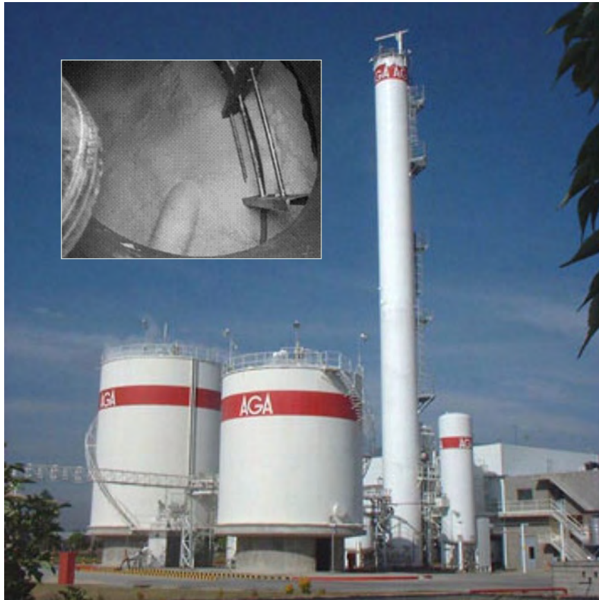
Figure 1-1. The cold box (inset) and the plant where two workers were asphyxiated by nitrogen
